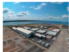
Haizea Breizh Offshore Towers Brest (France)
