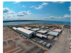
Haizea Breizh Offshore Towers Brest (France)
