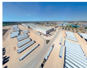
Haizea Tecnoaranda Onshore Towers Aranda de Duero (Spain)
