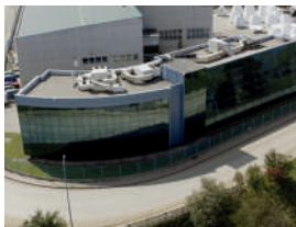
Haizea Grupo WEC (Machining and coating). Deba (Spain)
